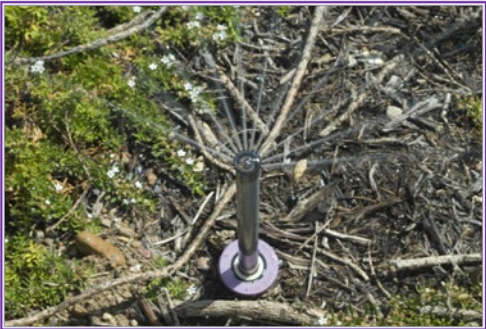
Purple is the standard color used to indicate that recycled water is in use at the site.
